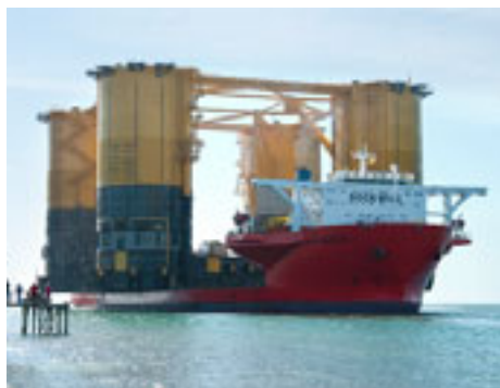
↑ The hull of the new platform for the Mars B project.
