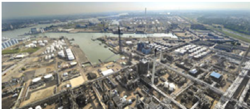
↑ Our Pernis refinery in Rotterdam, the Netherlands, has improved its energy efficiency.
